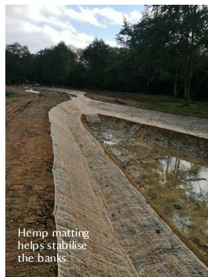
The swales and top edges of the ponds were lined with hemp matting to stabilise the
